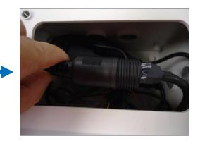
3. Secure the flex conduit fitting onto the junction box hole.
